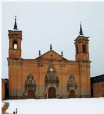
Main façade of the New Monastery
