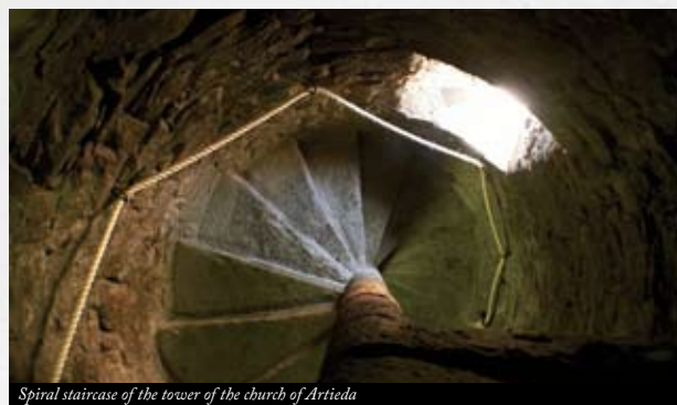
Spiral staircase of the tower of the church of Artieda
